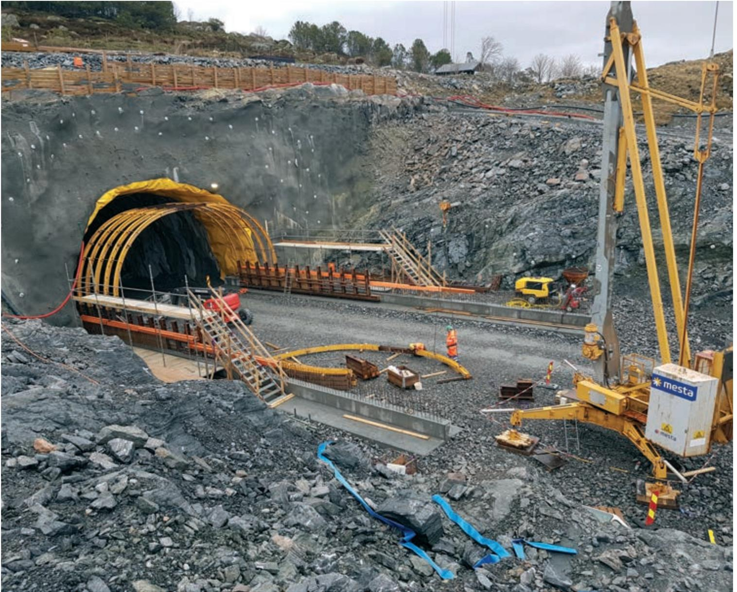
Formwork on the portal for the Haramsfjord tunnel from Hestøya is underway.
