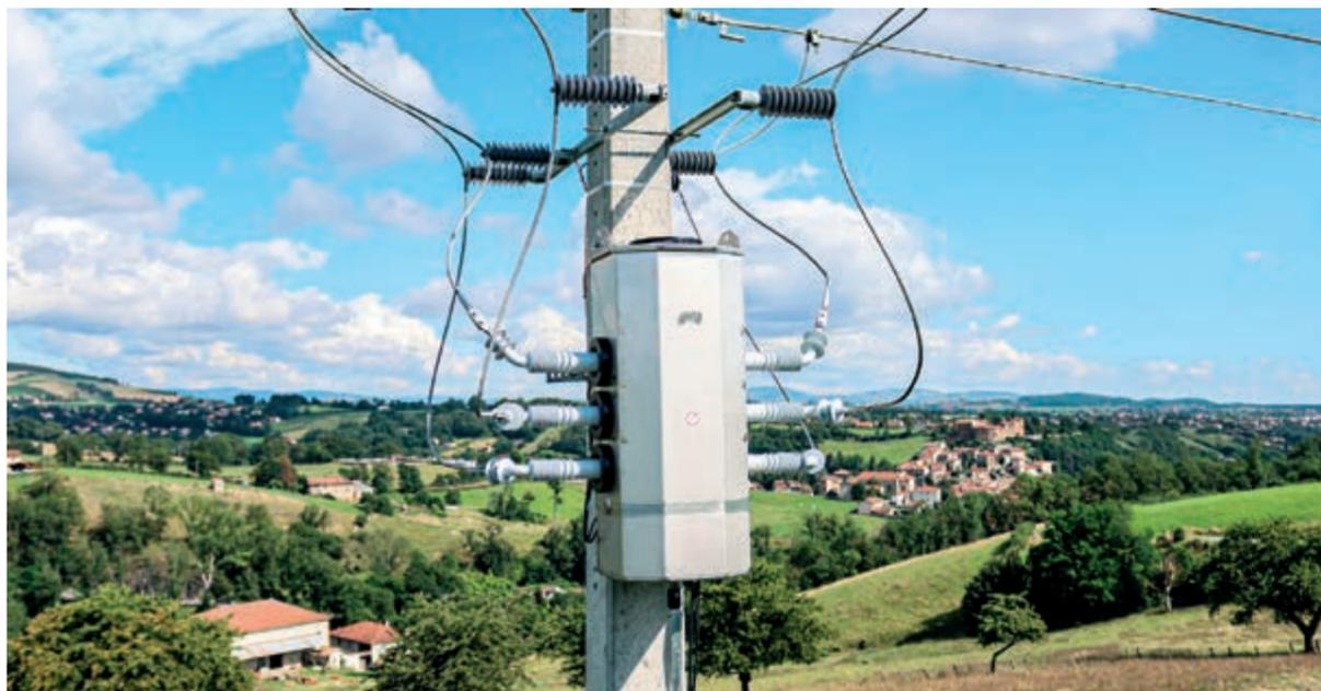
Auguste switch disconnecters isolate automatically a faulty part of a network and thus allows to re-energize all the remaining healthy network.
