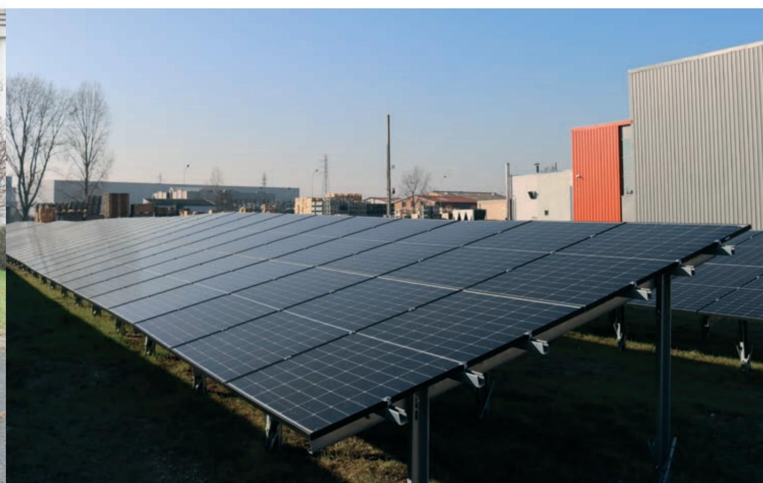
At left: Electric bicycles and their sheltered charging station. At right: Five hundred solar panels occupy 2,000 square meters, covering roughly 30 percent of the factory's needs for electricity.
